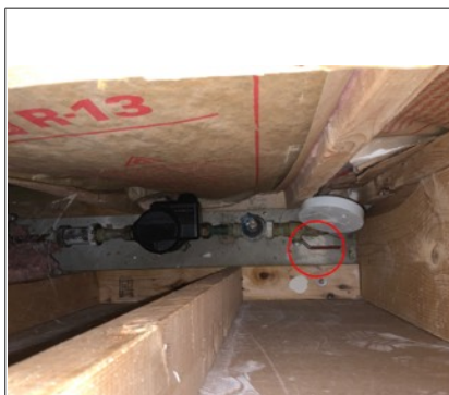
Main water shut off valve
