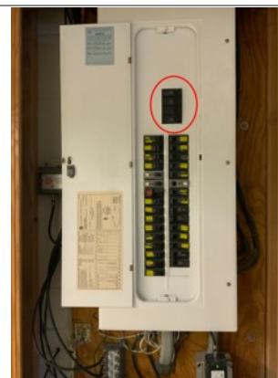
Main power disconnect location
