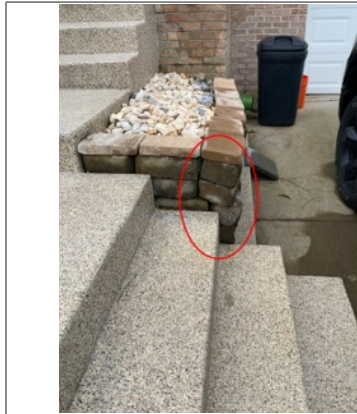
Retaining wall was leaning and had areas of separation at the block joints, recommend repair.
